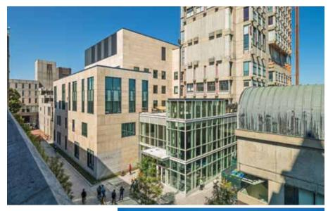
a practice court room, café, study and lounge spaces. In the second phase (scheduled to open August 2015), the architect restored the existing tower structure. Concrete and precast panels were repaired and window and metal panels were replaced with modern, energy-efficient assemblies of similar design. The total gut renovation of the interior provides new, updated offices for faculty, administration and student services.
