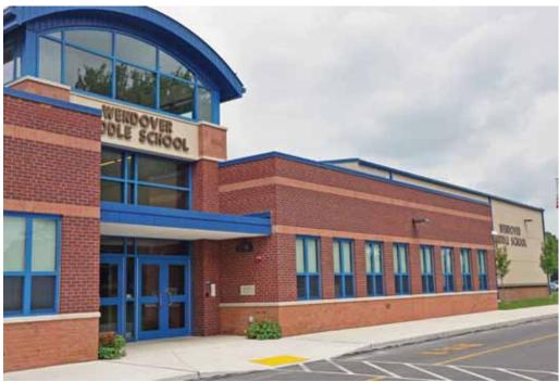
The Wendover Middle School is a steelframed, metal-sided building of approximately 98,000 sf, constructed in 1970. This construction project included 19,000 sf of additions, total replacement of all interior finishes and materials and selective demolition and construction. It also included a complete upgrade of the mechanical, electrical and plumbing systems. The existing
