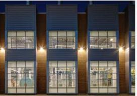
When BYU-Idaho became a four-year university, it had outgrown the 50-year-old coal-based plant used to generate heat for the campus since 1963. The university chose to upgrade to a highly efficient 5-bay facility with natural gas bollers and cogeneration unit, which now supplies over half the campus's power and steam requirement for heat. This essential facility provides students with a physical environment conducive to learning, regulating ambient thermal comfort consistently and efficiently.
